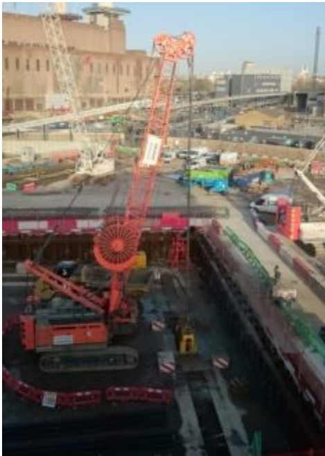
Figure 9: Excavation of a station box
