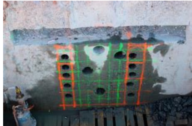
Figure 7: Core drilling in the D-Wall element of Producer II
