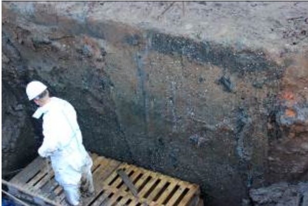
Figure 4: D-Wall element of Producer II after excavation
