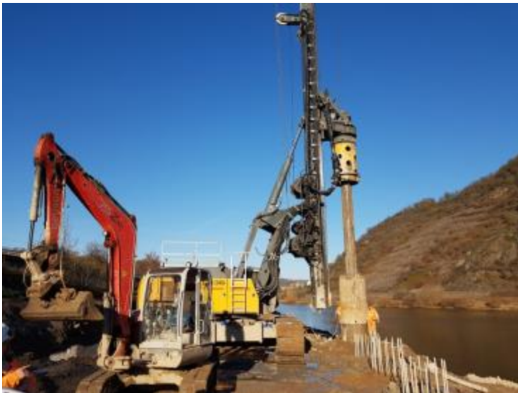
Figure 15: Bored piles for a new lock
