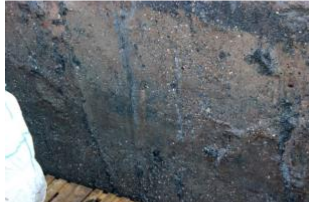
Figure 5: D-Wall element of Producer II after excavation (detail)
