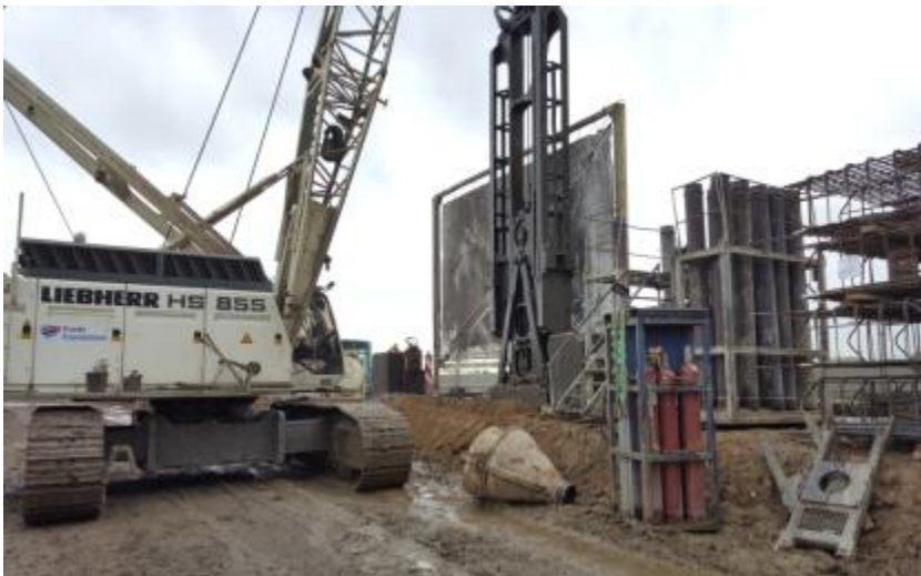
Figure 2: Excavation of a D-Wall element of Producer I
