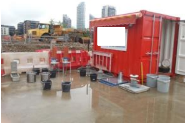
Figure 10: Testing area at the construction site of Producer III
