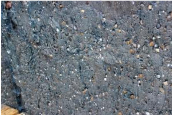
Figure 6: D-Wall element of Producer II after excavation (detail)
