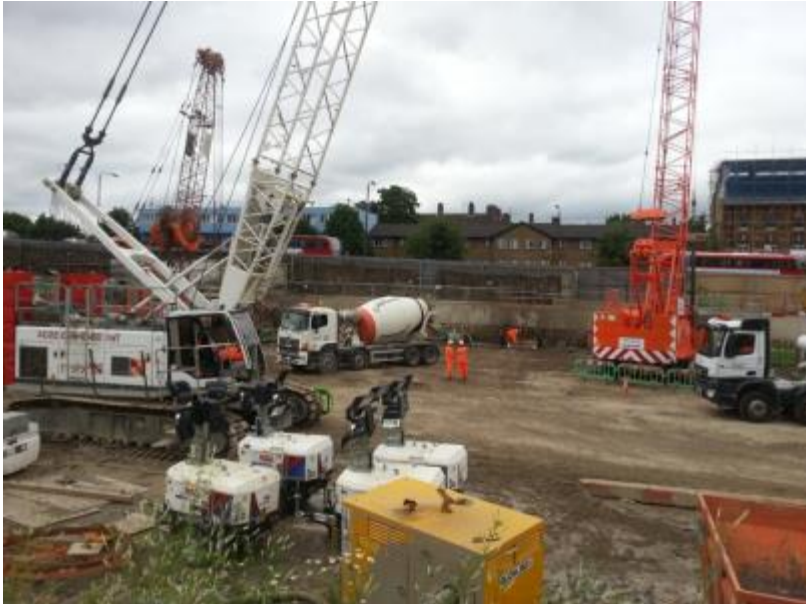
Figure 13: Concrete placement for a D-Wall panel
