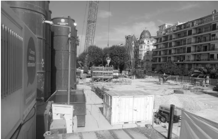
Figure 14: Construction site for a new station box for a future subway
