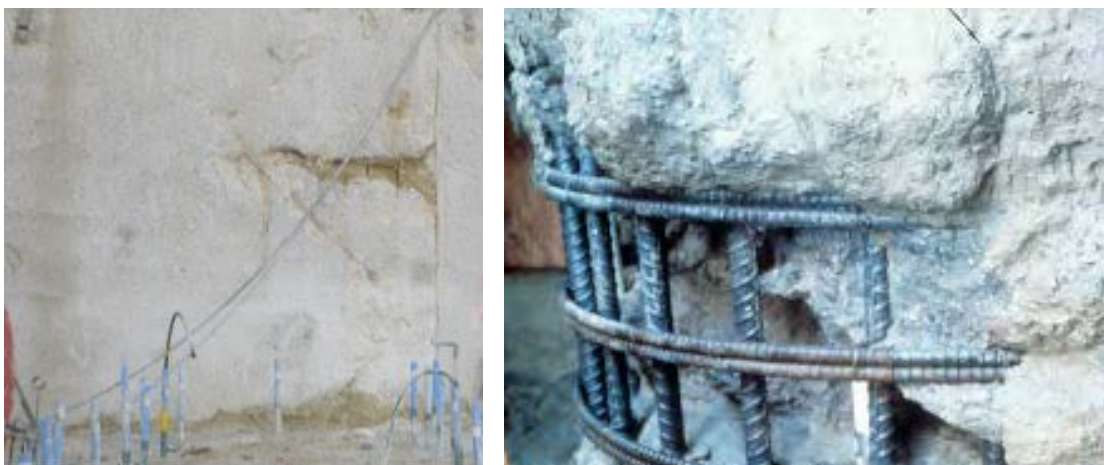
Figure D.2: Examples of inclusions of a diaphragm wall and a pile (pile photo taken from Figure 9.14b, FHWA GEC10)
