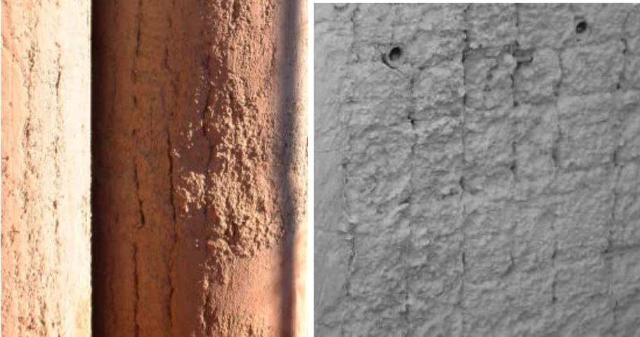
Figure D.4: Shadowing in a pile ( left ); matting in a panel ( right )
