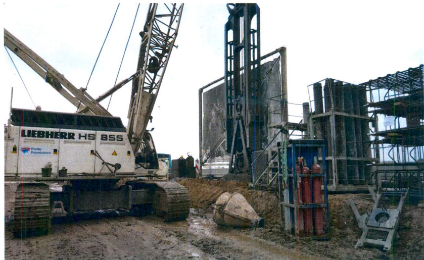
Figure 1: Excavation of a D-Wall element at Nieuw Lekkerland
