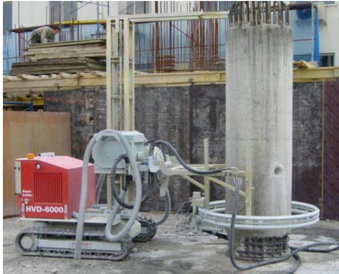
Typical Hydro-demolition Pile Breaker
