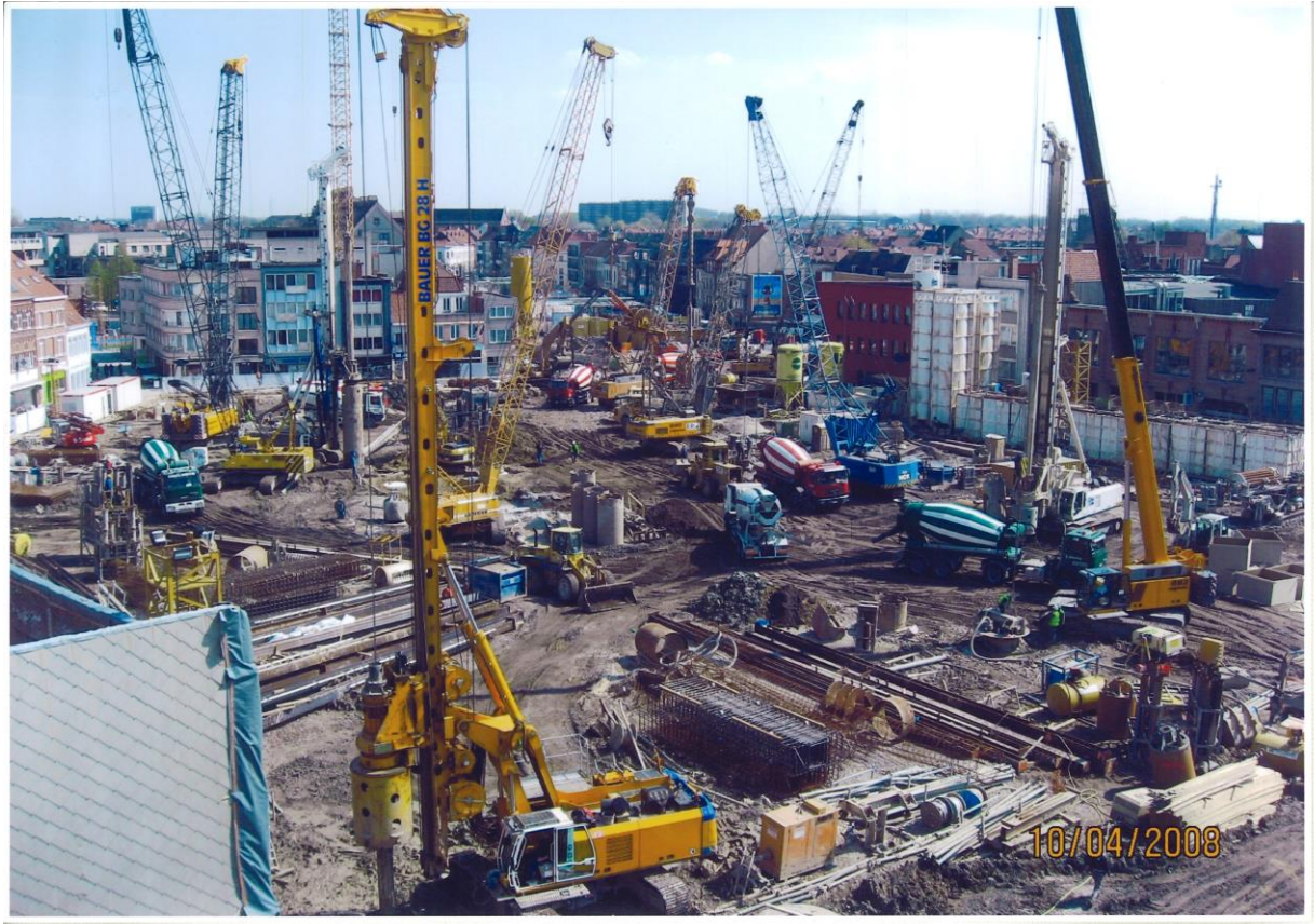
Fig 1: a busy site needs top quality safety management and co-ordination
